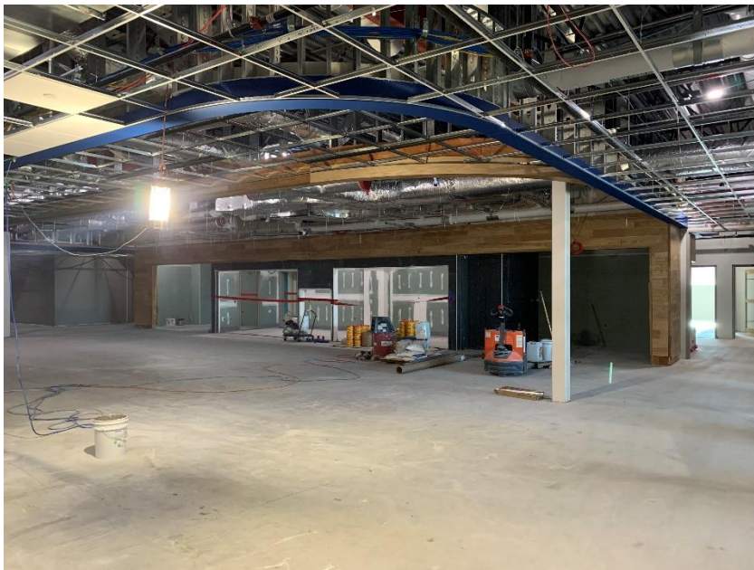
16. Area 3 – Wood plank install in second floor flex café in progress.
