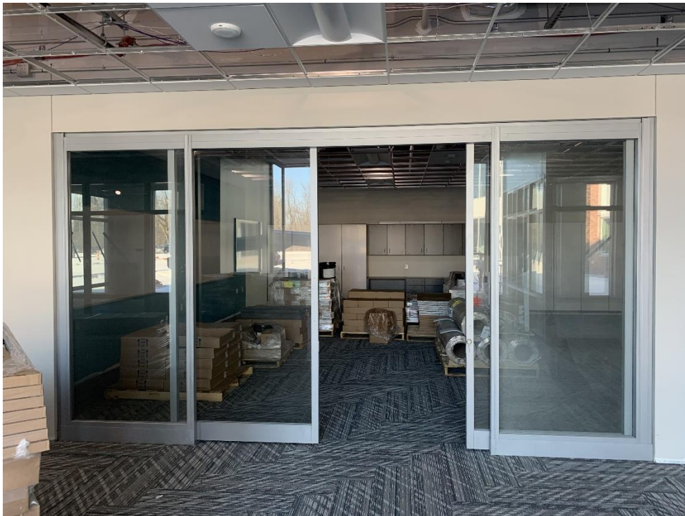
2. Area 6 – Classroom sliding door install in progress on both first and second floors.
