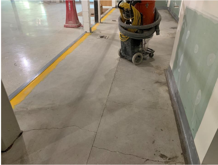
15. Area 5 – Epoxy floor install in second floor servery in progress.
