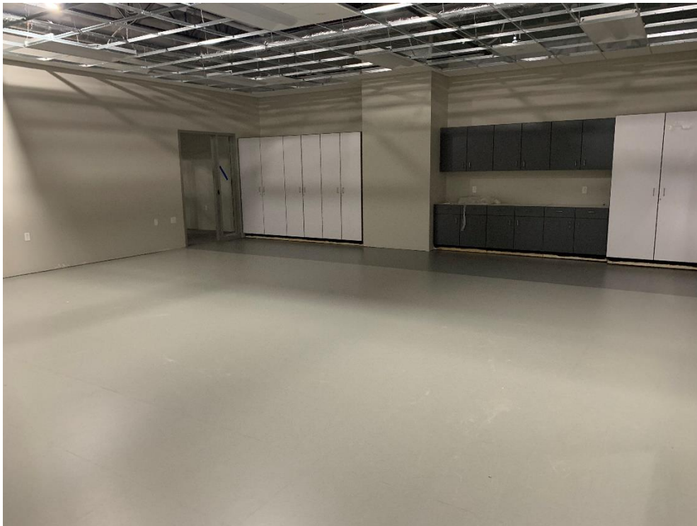
14. Area 6 – Resilient flooring in second floor EBD rooms appear to be installed.
